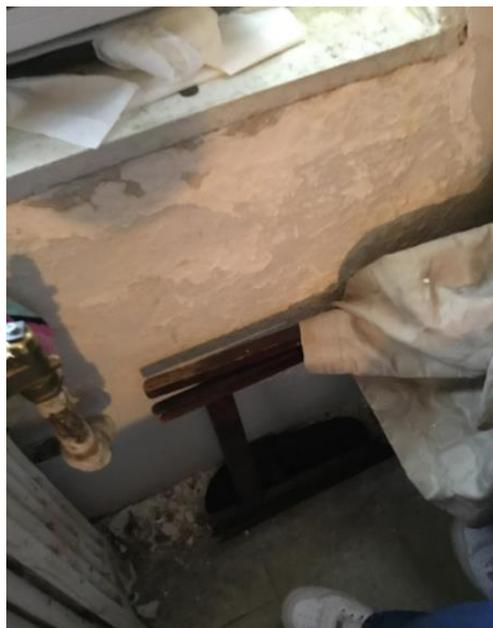
*Chipping paint in bedroom in the South Jamaica Development. Lead dust sample of 320  $\mu\text{g Pb}/\text{ft}^2$  – Queens*
